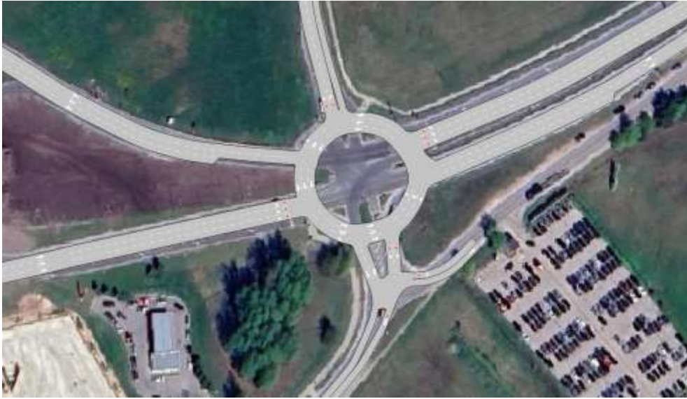
Figure 16 – Intersection turned into a roundabout Source: Ineco
